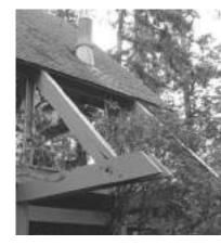
The exposed rafters and joists of the A-frame design have led to rot issues around bolted joints Photo by Dale Kutzera
